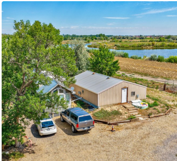
Private wastewater treatment facility
